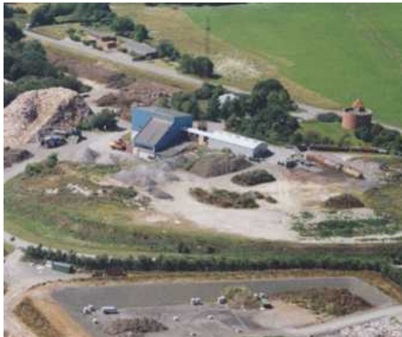
The Oil and Hazardous Waste Station
